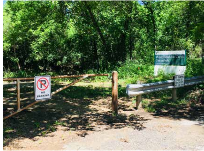
Zone 1. View of existing signage at service entrance w/ metal access gate, bollard and guardrail.
