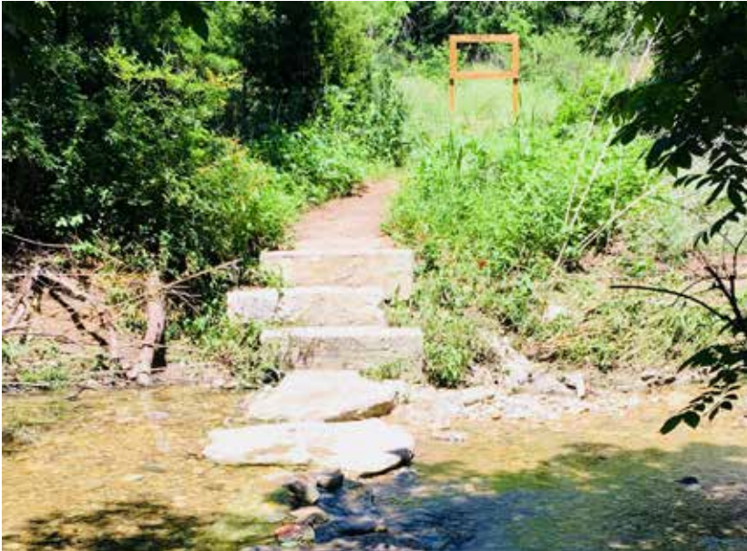
Zone 3 Rock hop and limestone steps across creek bed to trails
